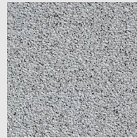
CT-6 Ceramic Tile Service Floor, Service Reception
