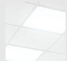
ACT-4 Acoustic Ceiling Tile Service Reception
