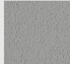
EIFS-2 Exterior Insulating Finishing System, Exterior Rear Facade
