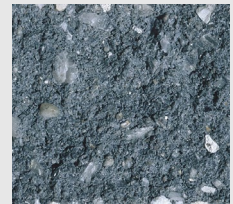
CMU-1 Concrete Masonry Unit, Exterior Perimeter of Building
